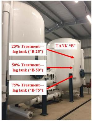
Figure 1—Kroll Well GAC Treatment System Sampling Locations
